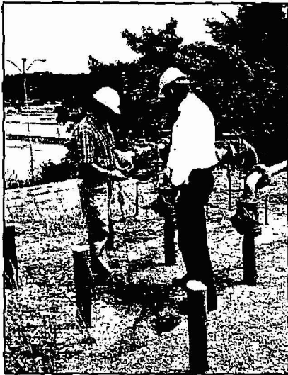
Staff members John Amerman and Bob Leonberger checking the corrosion protection level on the pipeline.
