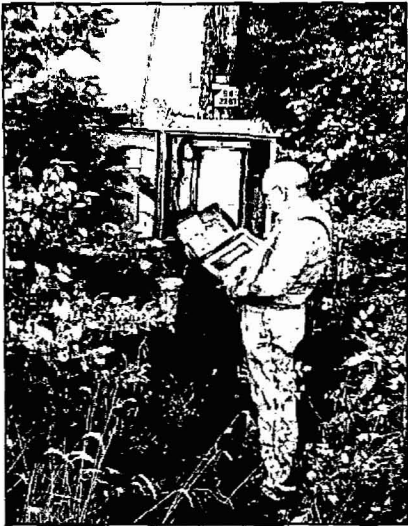
PSC staff member Myron Couch analyzing the effects of a recently installed telephone company Power Influence Neutralizing Transformer.
