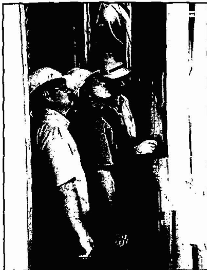
PSC engineers Leon Bender and David Elliott inspecting a boiler at KCPL's Hawthorne power plant.
